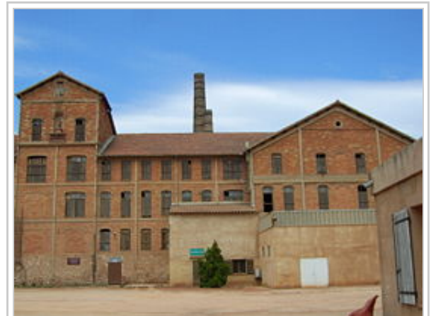
Building which served as a concentration camp at Camp des Milles.
